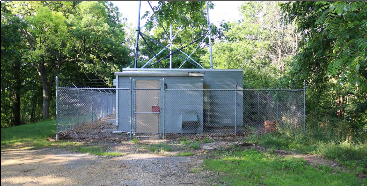
Photo 2 - COMPOUND OVERVIEW—LOOKING SOUTH
