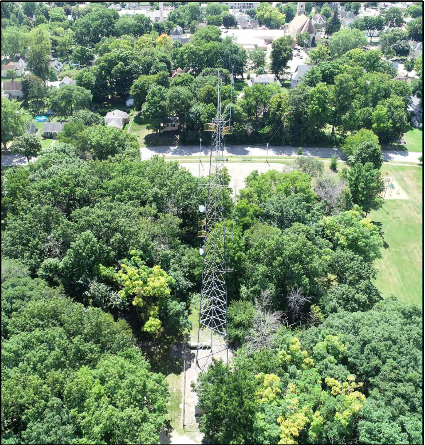
Photo 1 - EXISTING TOWER OVERVIEW
