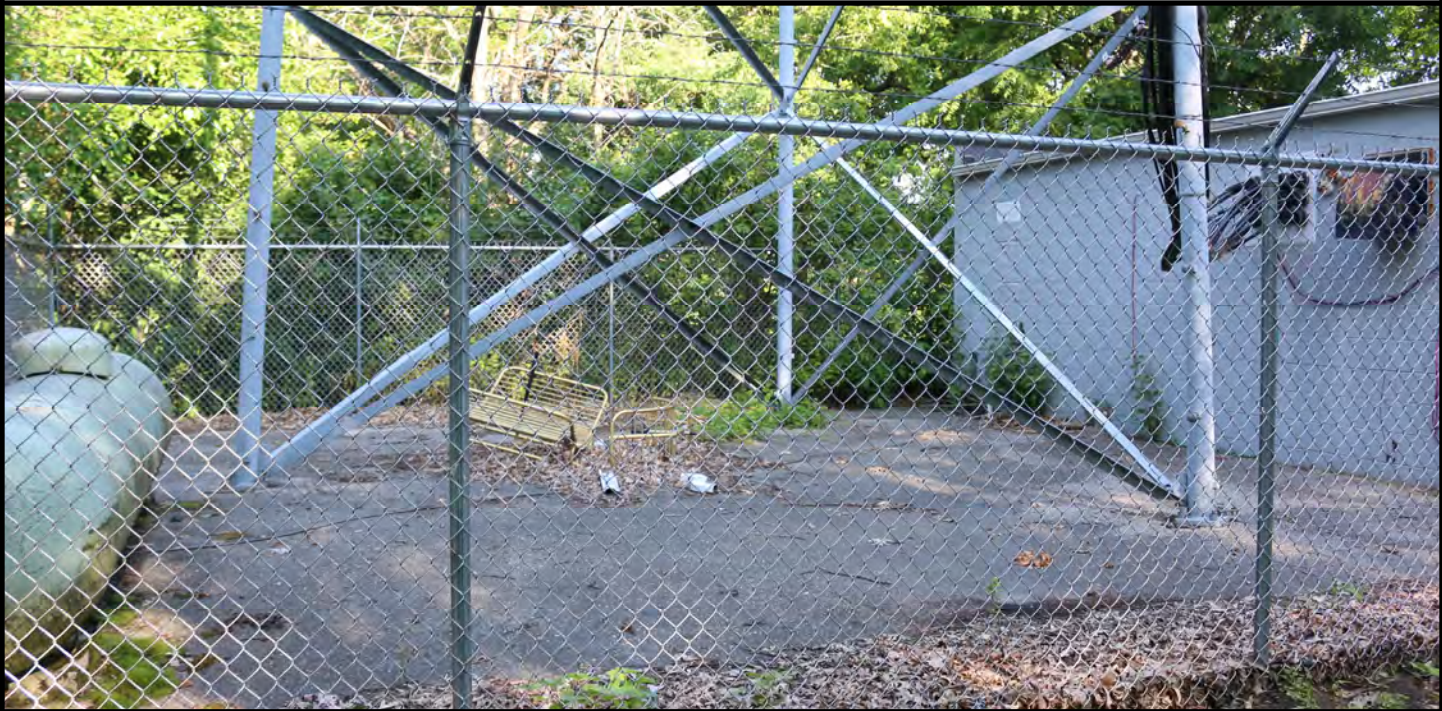
Photo 3 - EXISTING TOWER BASE
